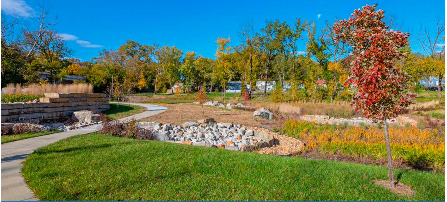
Green infrastructure helps our community manage stormwater the way nature intended by capturing and utilizing rainwater where it falls. The Rachel Morado project, located in south Kansas City, absorbs and filters 500,000 gallons of stormwater from approximately 82 acres in the Middle Blue River Watershed Basin.
