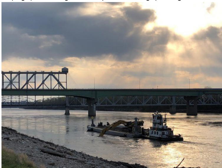
A backhoe on a barge pushed by towboat performs maintenance on a levee by Berkley Riverfront on the Missouri River.
