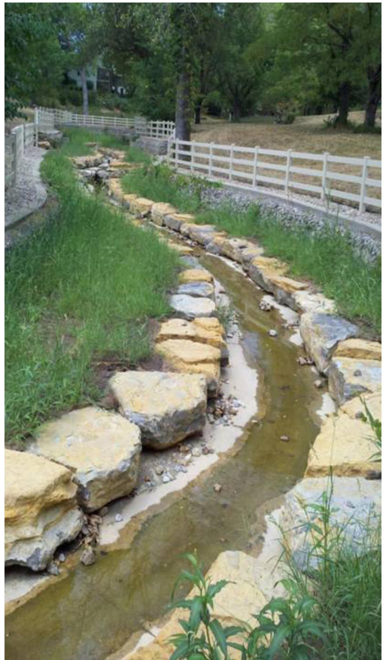
Stormwater improvements include rock-lined channels in neighborhoods.
