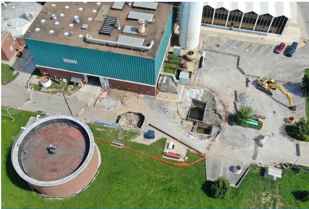
Excavation work has begun for a new biosolids treatment facility that will end incineration and instead produce useful fuel and fertilizer at KC Water's Blue River Wastewater Treatment Plant.
