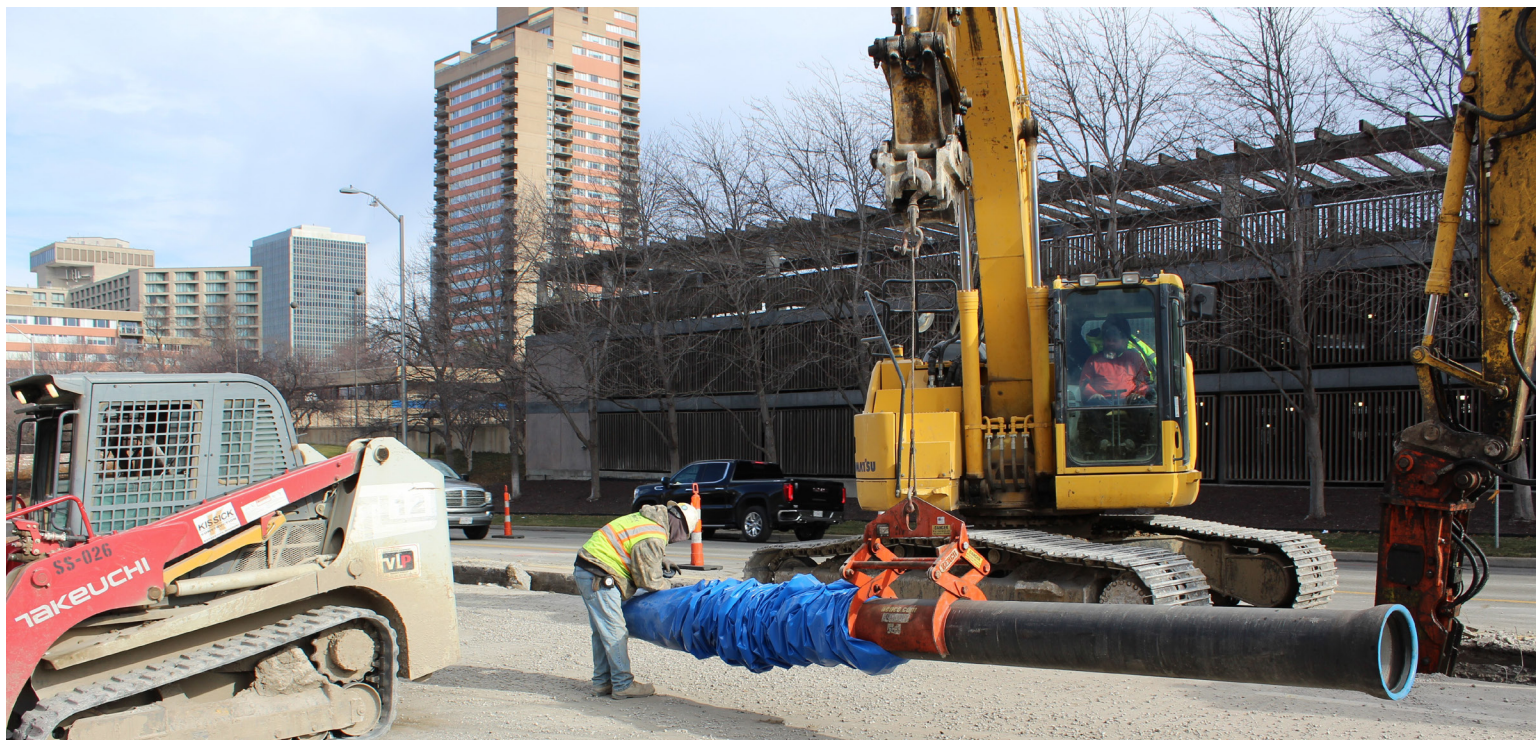
Ductile iron pipe is wrapped in thick polyethylene before being buried near 27th and Main streets as part of the Upgrades on Main project.
