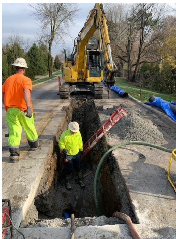
A trench on State Line Road near 55th Street is readied for a new water main. Water mains are installed deep enough to prevent freezing during winter.
