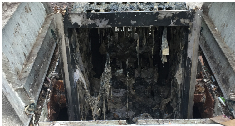
Wipes not only clog wastewater treatment equipment, but they also may block home and neighborhood sewer lines. Never flush wipes.
