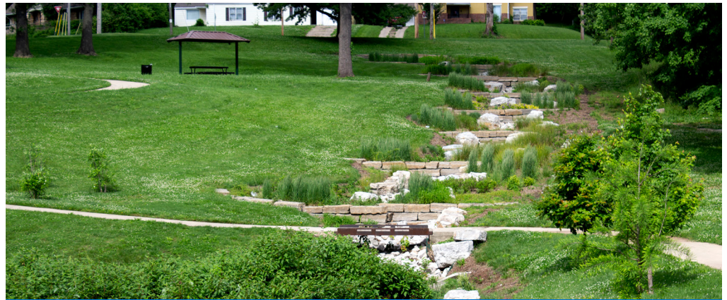
Arleta Park at 77th Street and Prospect Avenue in the Marlborough neighborhood of south Kansas City is an example of green infrastructure that improves stormwater drainage while beautifying a neighborhood asset.
