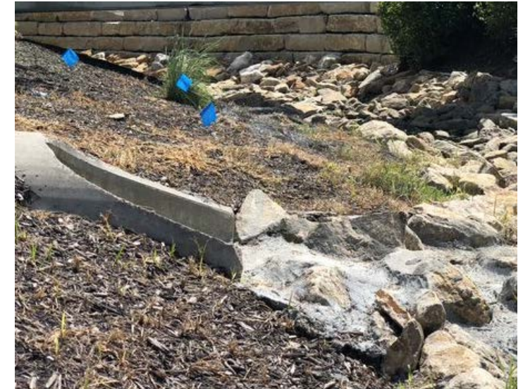
2.1 Concrete Embedded Splash Pad
