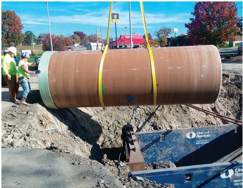
An 84-inch fiberglass pipe was used to replace a rusted corrugated metal pipeline on Eastwood Trafficway this fall.
