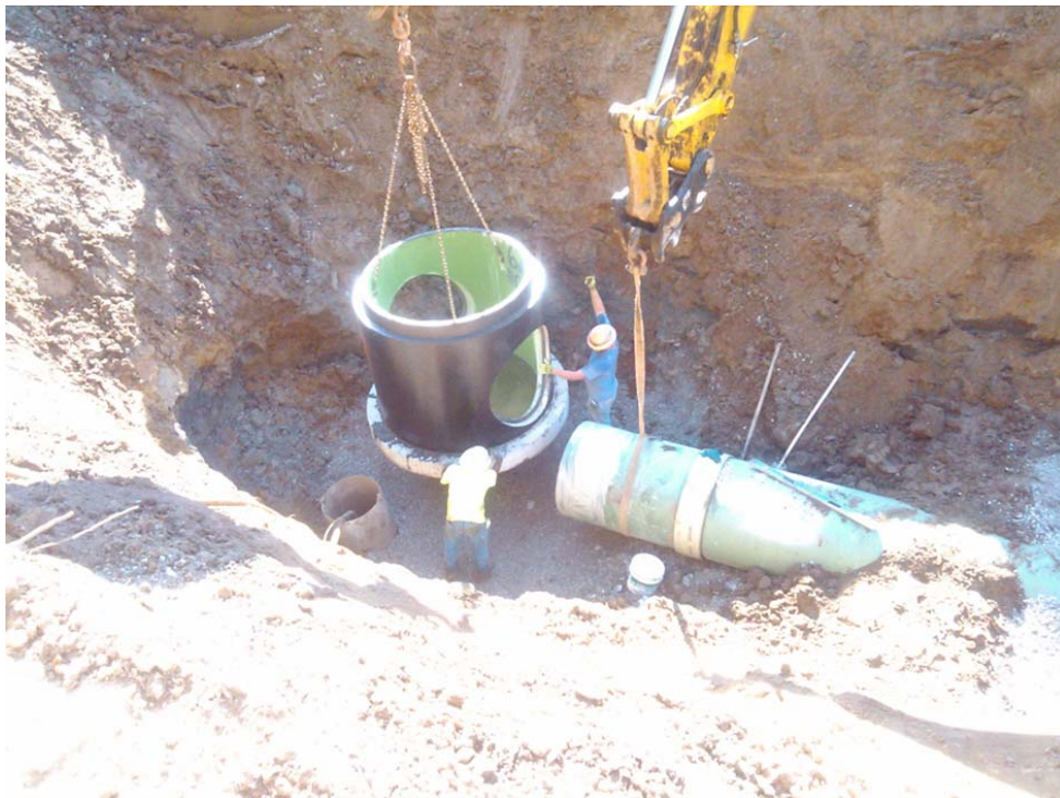
Connection to new manhole on 36-inch diameter pipe
