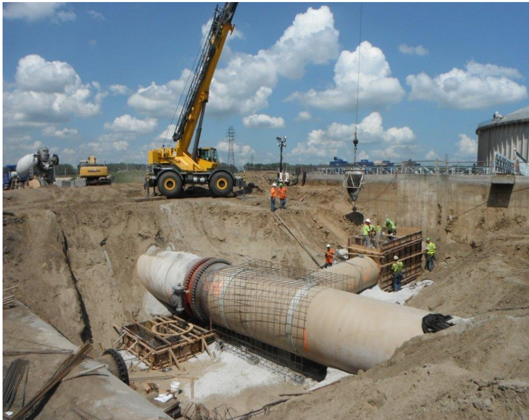
Blue River: Connection of the New 96" Effluent Discharge Line to Clarifier No. 4
