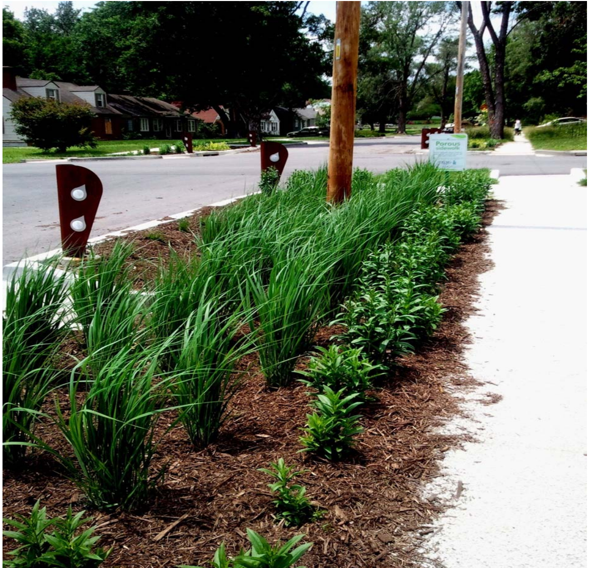
Curb Extension w/Rain Gardens at 75th Terrace and Lydia (looking west)
