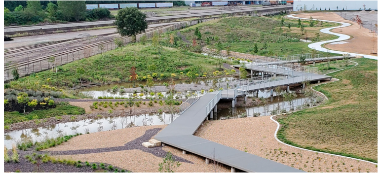
A green space in the West Bottoms that allows rainwater to soak into the ground also includes a boardwalk and a public trail.
