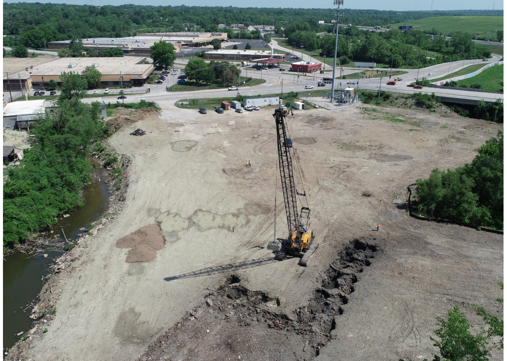
A 16-ton crane dropped a 19-ton steel weight from 60-feet in the sky in order to build a levee to protect the Dodson Industrial District from flooding. Compacting soil in the area will mean the levee can be built on a firm foundation without moving material.
